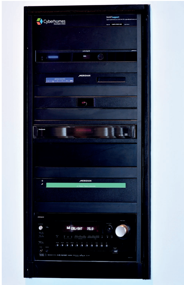
Dedicated AV rack is inset into the bespoke joinery built by Cyberhomes in-house fabrication team.
