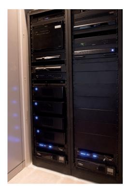
Two full height AV racks house all the centralised AV equipment with capacity for expansion.
